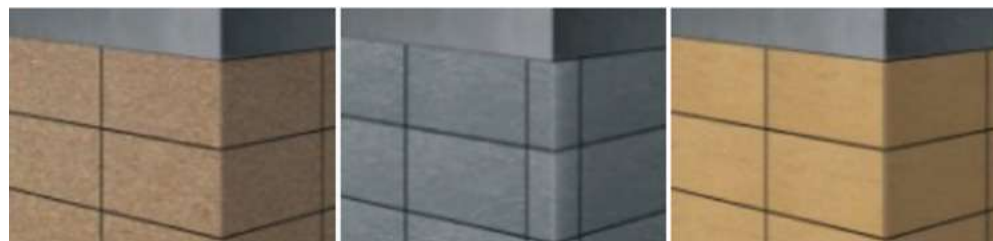
Butt joint primary color caulking
