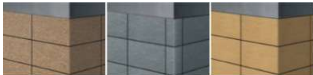
Butt joint primary color caulking
